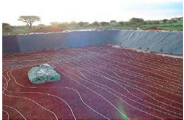
Figure 1. Photo Digester pit.
