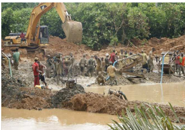
Fig 3. The small-scale mining activities undertaken along the river bed in denawase, Ghana
